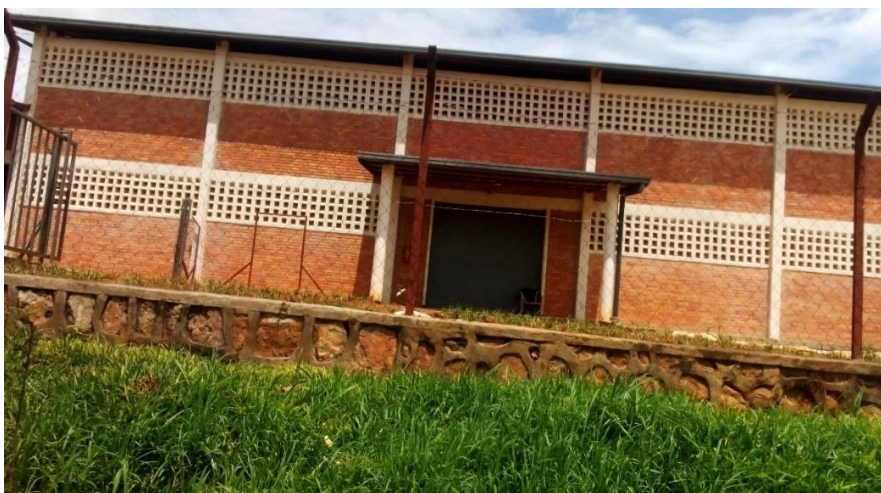
Figure 16: Storage facility built by MINAGRI in Nyabugogo village for COOPAMA Cooperative
