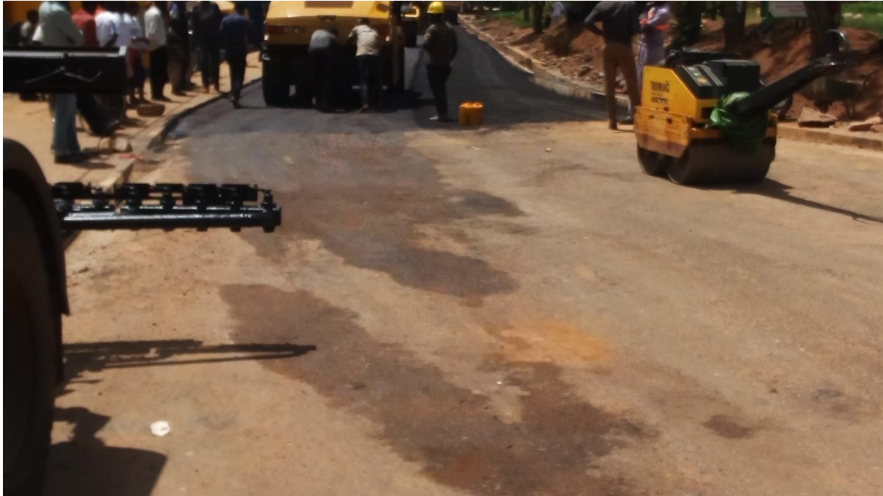
Picture 4: Ongoing road construction in Nyagatare
