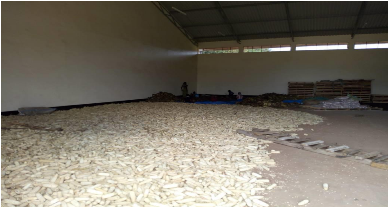
Figure 6. Picture of the warehouse constructed at Babati
